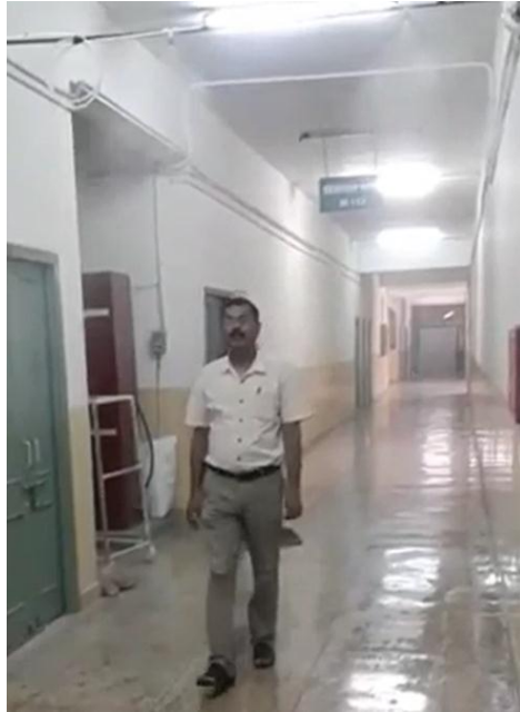
Fig. :- Automatic Sanitizer Spray Facility
